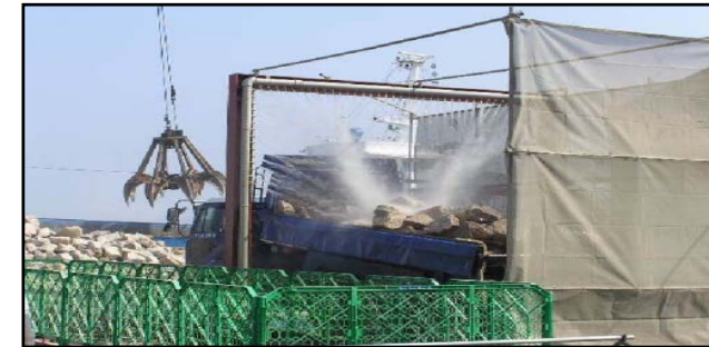
Flushing of rubble
